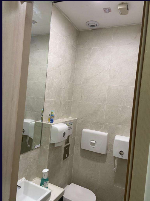
Toilet @ CIC office
